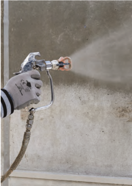
LEFT, BELOW AND BELOW LEFT: Mapei's Planiseal WR 100 hydrophobising liquid helps to prevent degradation and detachment of concrete. The system can be applied by spray or roller.
