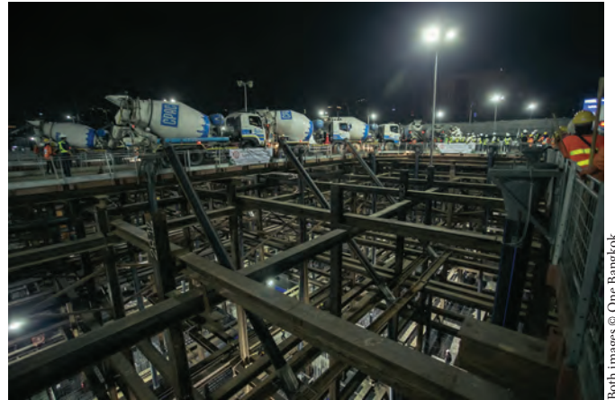
ABOVE AND LEFT: The raft foundation pouring for one of the office towers at One Bangkok has been completed. It involved the coordination of 547 trucks, providing a total of 23,725 cu m of concrete.
