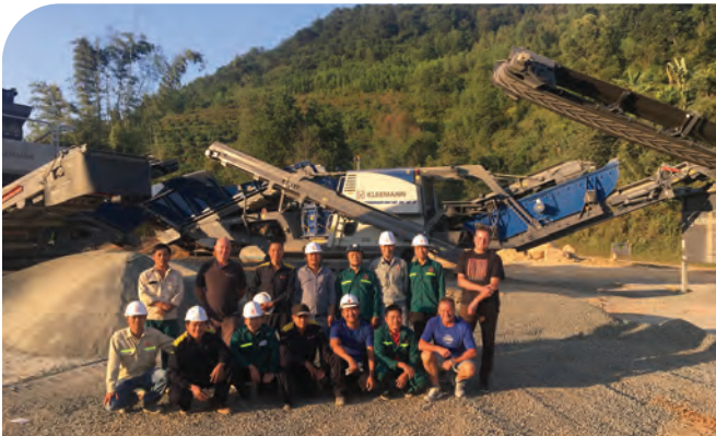
Licogi 16 JSC is carrying out a number of road and bridge construction jobs on the National Route 1A project. To help with the work, the company opted for a track-mounted interlinked plant combination from Kleemann.
