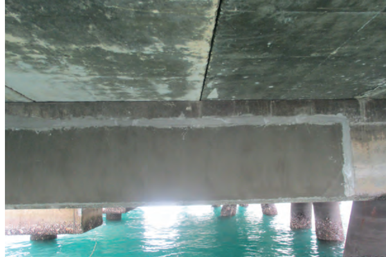
ABOVE (LEFT AND RIGHT): Mapei's Planiseal WR 100 and Planitop Smooth & Repair R4 systems were recently used to help repair a jetty structure on one of the southern islands in Singapore.
