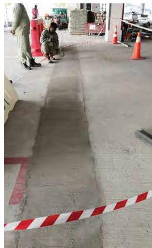
BELOW (LEFT, MIDDLE AND RIGHT): The Planitop Smooth & Repair R4 cementitious mortar has also been chosen for carpark floor repair at the Airbus Training Centre in Singapore.
