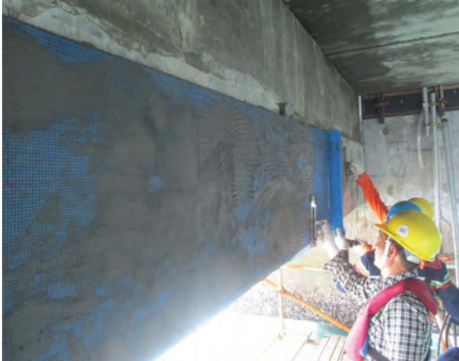
ABOVE (LEFT AND RIGHT): Mapei's Planiseal WR 100 and Planitop Smooth & Repair R4 systems were recently used to help repair a jetty structure on one of the southern islands in Singapore.
