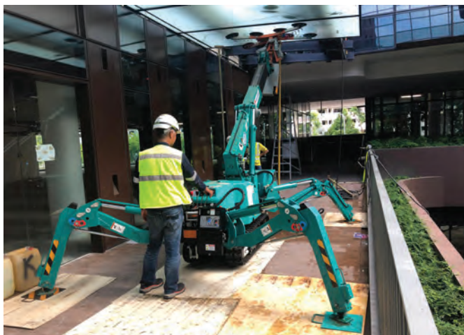
ABOVE: The Oktopus vacuum lifting device being used together with a Maeda mini crawler crane (spider crane) to perform glazing work on a construction project in Singapore.
