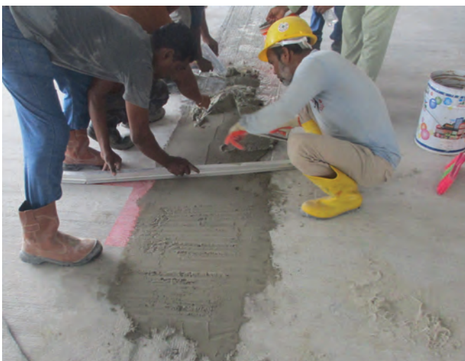
BELOW (LEFT, MIDDLE AND RIGHT): The Planitop Smooth & Repair R4 cementitious mortar has also been chosen for carpark floor repair at the Airbus Training Centre in Singapore.
