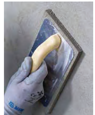
LEFT, BELOW AND BELOW LEFT: Mapei's Planitop Smooth & Repair R4 system is designed for structural repairs. This cementitious mortar can harden without shrinking and features strong adhesion to concrete substrates.
