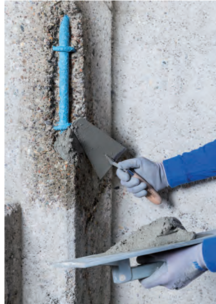
LEFT, BELOW AND BELOW LEFT: Mapei's Planitop Smooth & Repair R4 system is designed for structural repairs. This cementitious mortar can harden without shrinking and features strong adhesion to concrete substrates.
