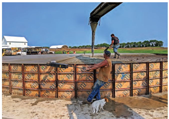
ALL IMAGES: The Batt Screed 6000 roller screed in action.
